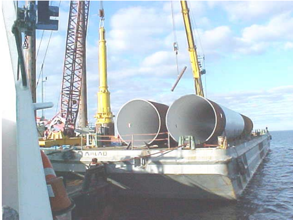
Figure 1: Jack-up Wind and Barge Bolle VIII with monopiles (Utgrunden)
