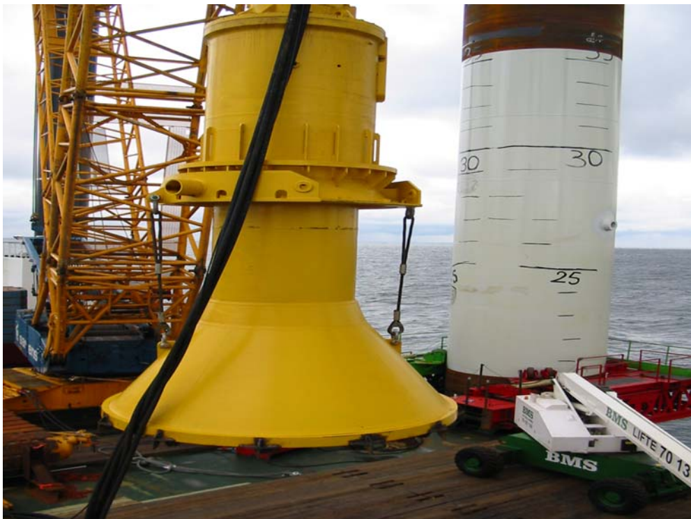
Figure 4: Jack-up Vagant and monopile in piling frame with hammer MHU 500 (Samsø)
