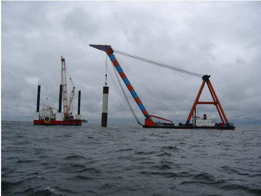
Figure 3: Hammer MHU 500 and piling adaptor diameter 4.5 m (Samsø)
